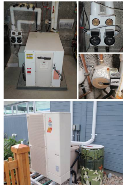
Figure 2: Ground source (top) and air source (bottom) heat pumps
